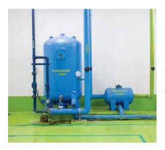
In a process heater system, an expansion tank serves a vital role in managing the thermal expansion of the heating fluid. Here's a break down of its purpose and function:
